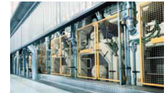
▲ View of the pre-dryer section with vacuum rolls and web stabilizers.
