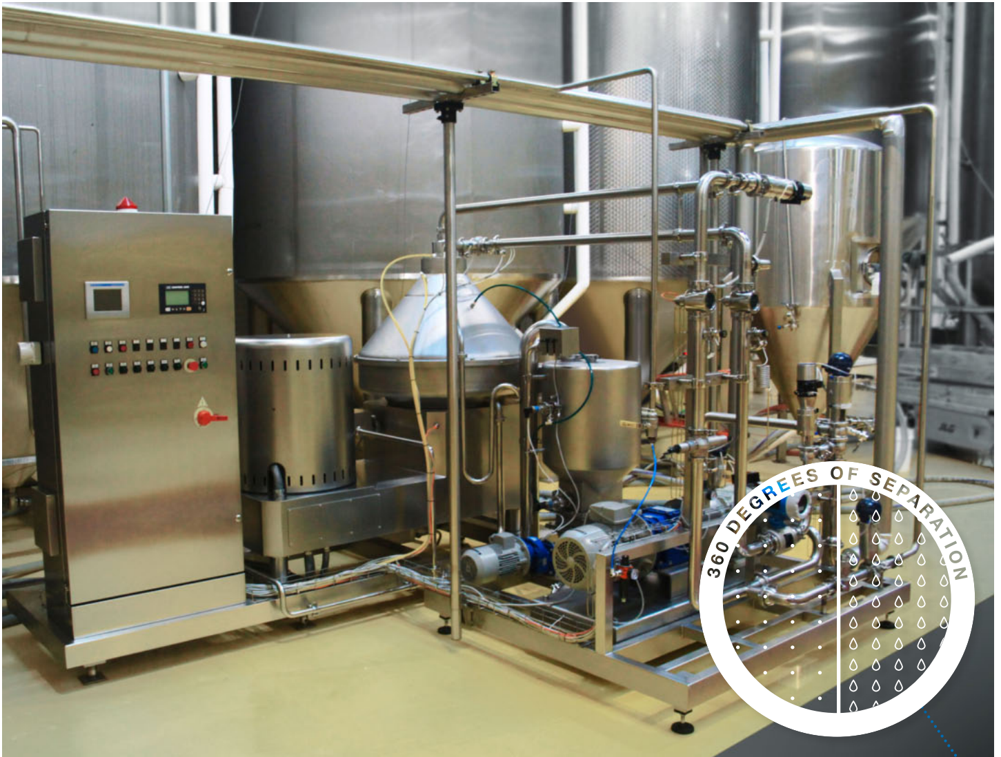
▲ Beer clarifier skid at Florida Beer Company production facility
