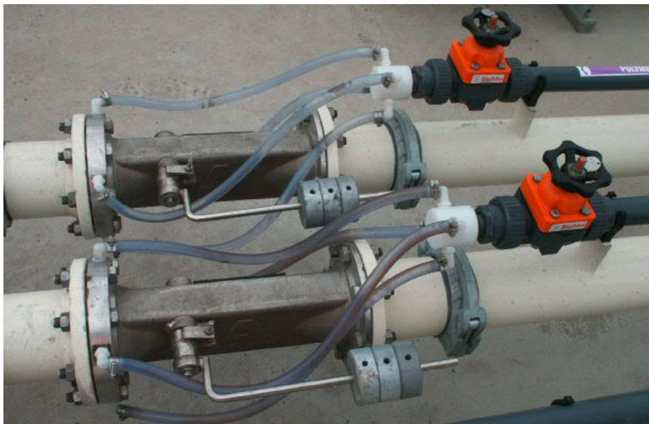
▲ Venturi mixer, inline flocculation system
