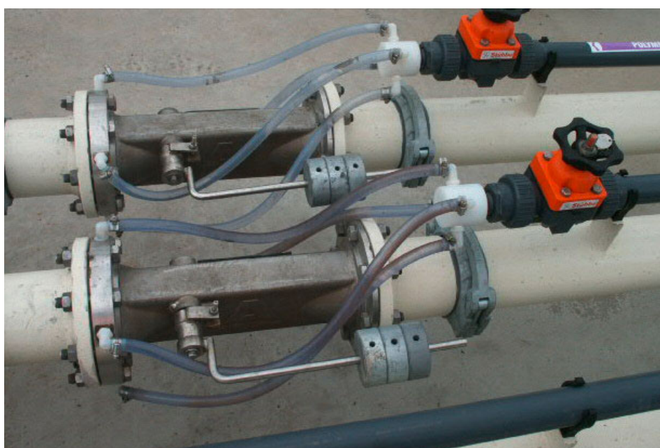
▲ Venturi mixer, inline flocculation system
