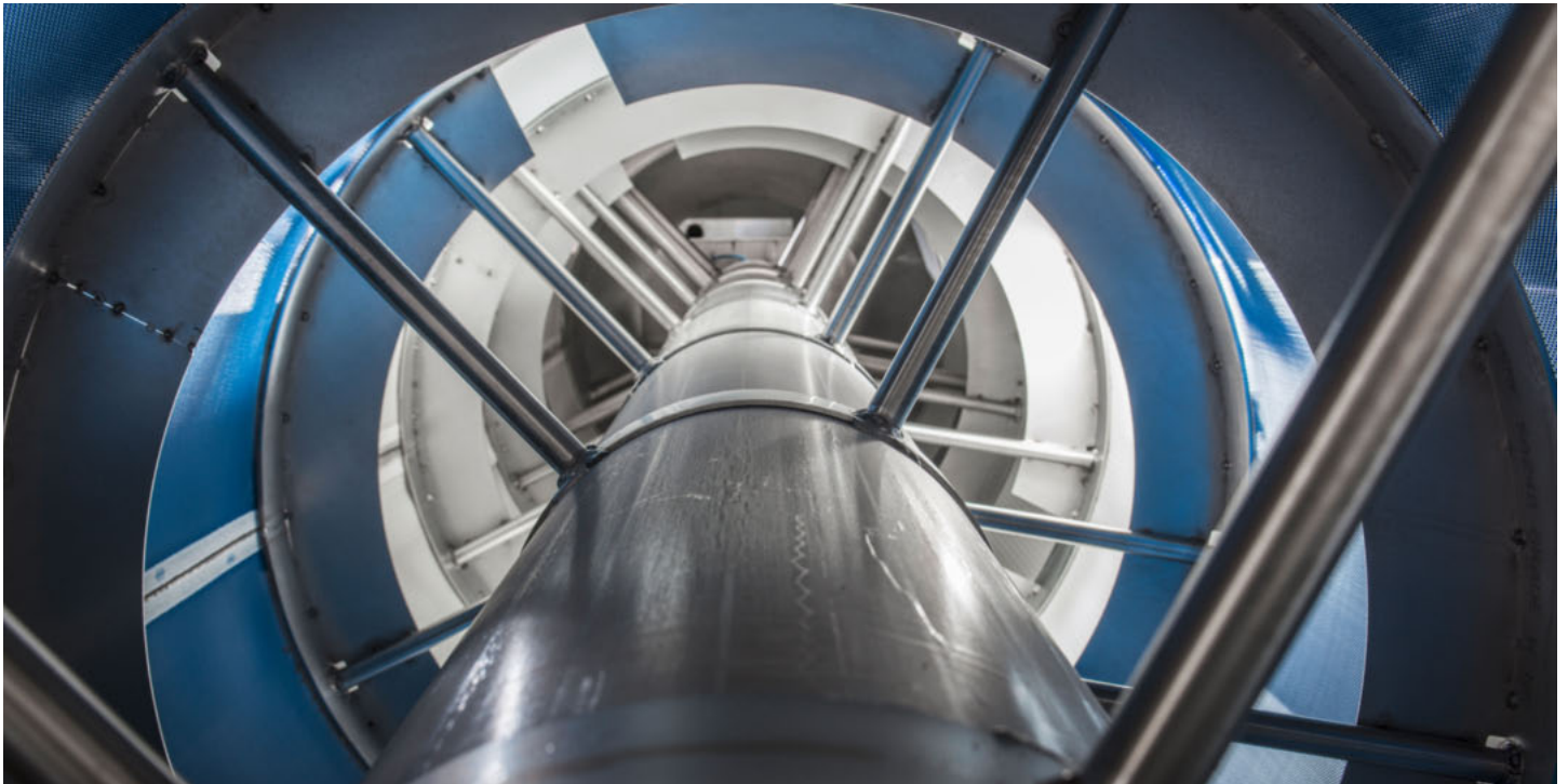
▲ Reliable technology allowing a significant reduction in sludge volume (up to 90%)
