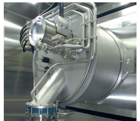
▲ Clean room installation
