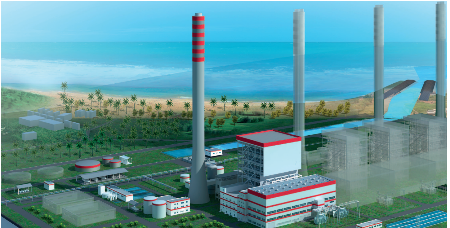
▲ Seawater FGD plant in Venezuela
