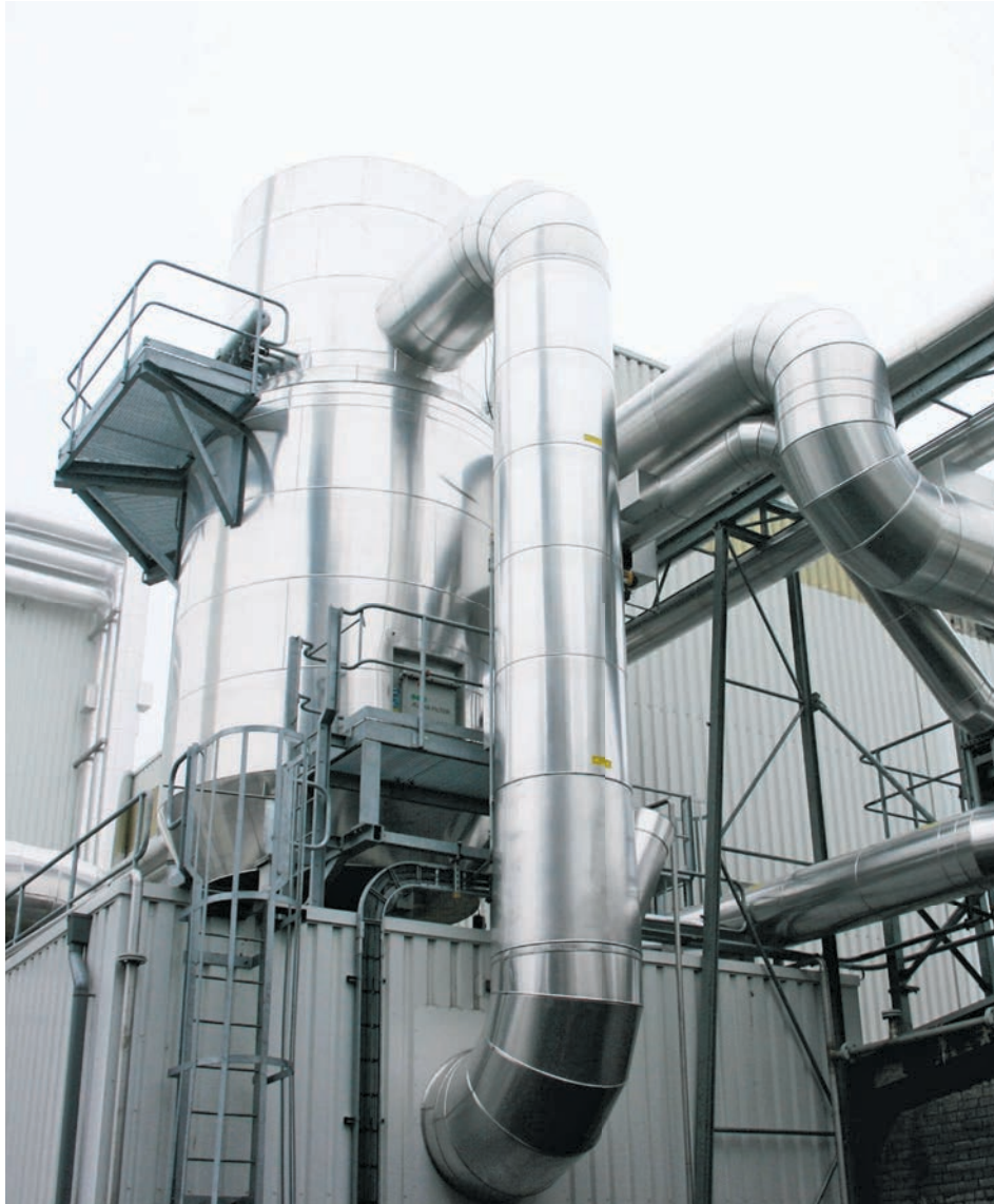
▲ Filter type DFAK Compact bag filter in rectangular housing and cleaned by compressed air. Used especially for mounting directly on screw conveyors, bucket elevators, and silos. Design: Horizontal or vertical Filter area: 1.8-5.4 m 2
