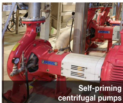
Single-stage centrifugal pumps Semi-open and open impeller
