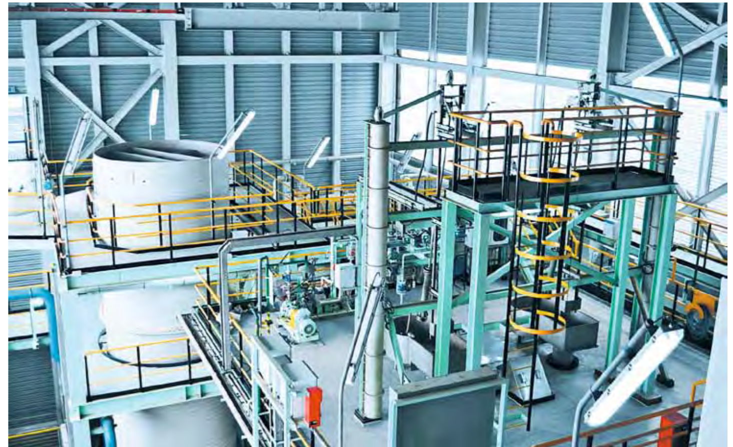
▲ PYROMARS reactor acid spray system, Malaysia
