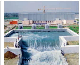
Kalwakurthy Stage 2, India Large pumps (5 × 30 MW, 5 × 23 m³/s) for agricultural irrigation in Andhra Pradesh 2016
