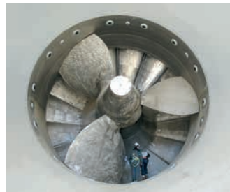
Sihwa, Korea Electro-mechanical equipment including 10 bulb turbines (26 MW each) for the world's largest tidal power plant 2006
