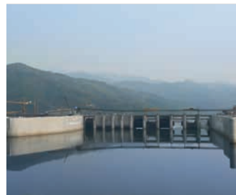
Xayaburi, Lao PDR Electro-mechanical equipment for the largest hydropower plant on the Mekong River in Lao PDR 2013
