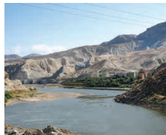
Ilisu, Turkey Electro-mechanical equipment for the largest hydropower plant in South-eastern Anatolia 2008
