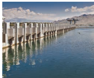
Ashta, Albania 90 modules for the world's largest HYDROMATRIX® power plant (Ashta I with 24 MW, Ashta II with 45 MW) 2008
