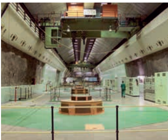
Ruacana, Namibia Turbines for Namibia's largest hydropower plant 1974
