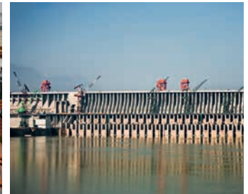
Three Gorges (Sanxia), China Turbines and generators for the world's largest hydropower plant 1997
